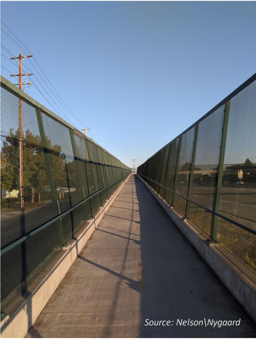
Bike and pedestrian bridges
