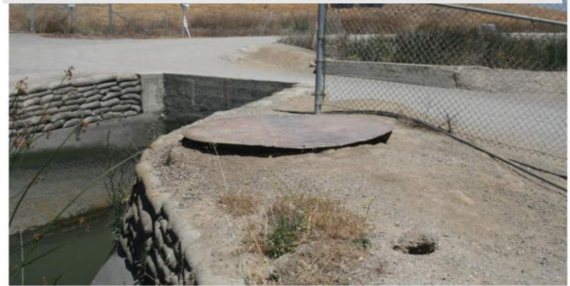
Carl Road Box Culvert at Sunnyvale West
