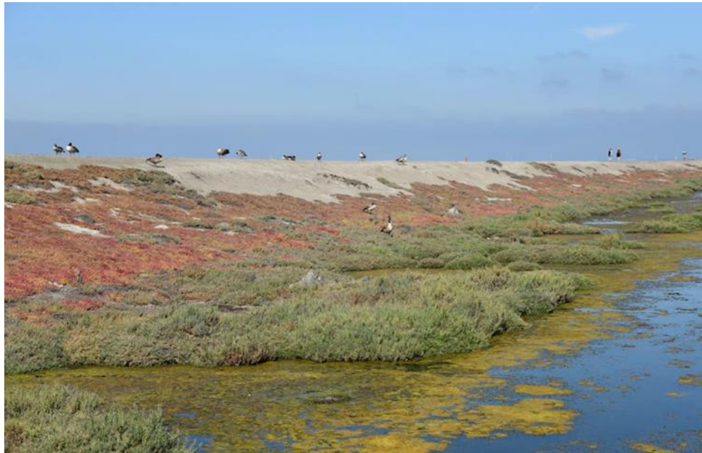
Existing Alviso Levee By Nick Simeone
